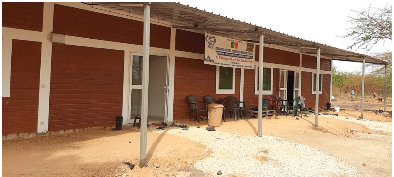
BELOW: Building constructed using a clay block press.
